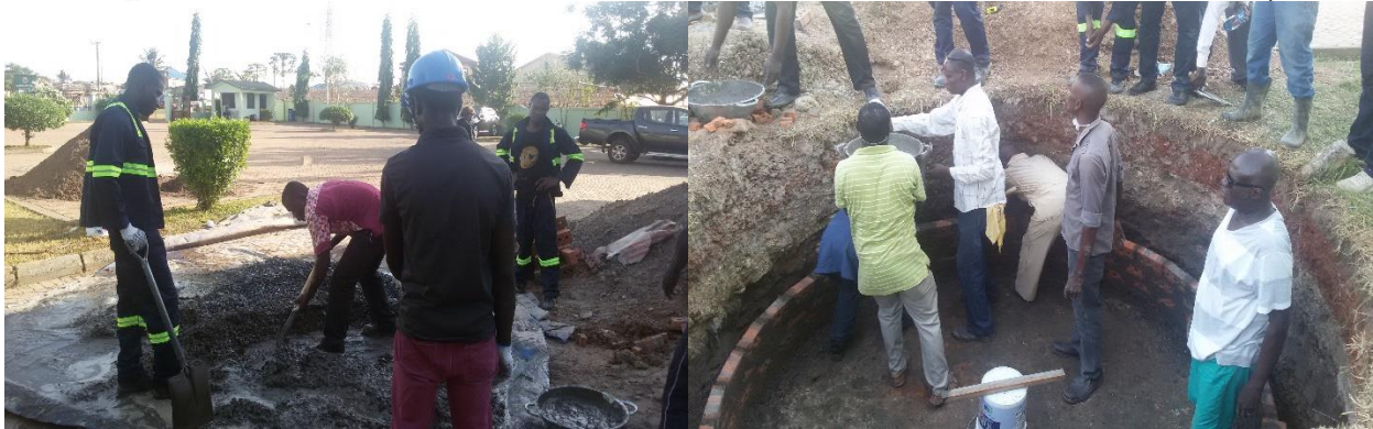
Mixing of concrete and laying of bricks
