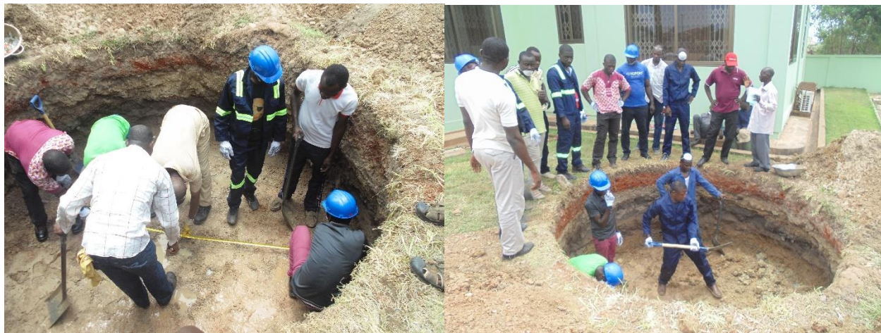
Setting out to commence
